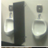
Pedregal Convention Center
